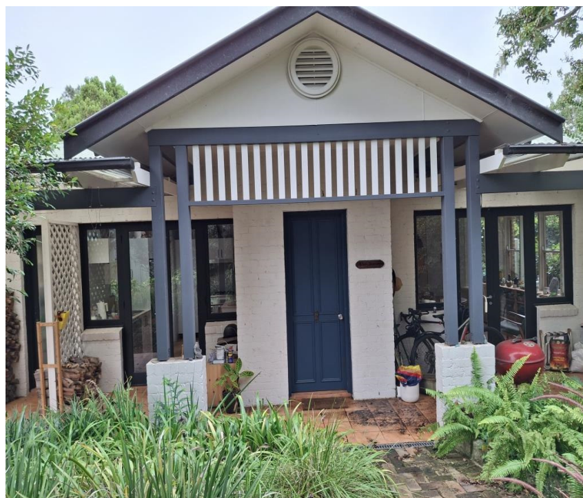
Rear entry of the existing house (to be demolished).
