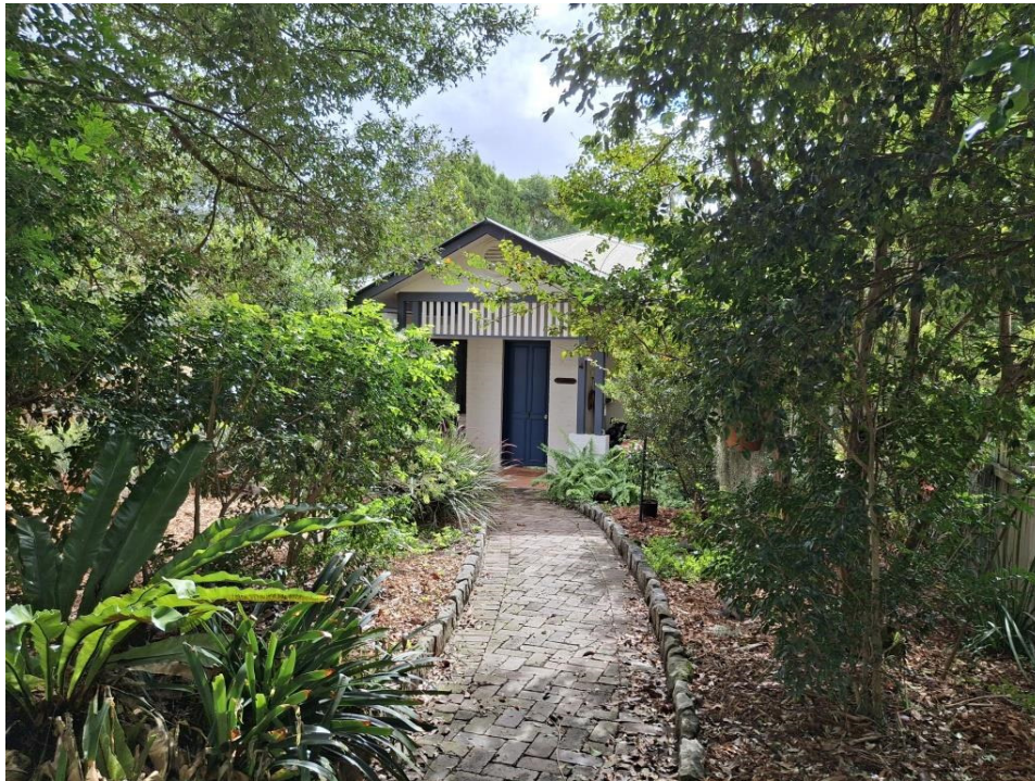
Entry path to the rear door.
